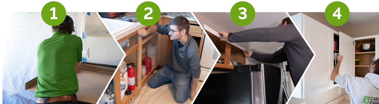
1 Removal of old doors and drawers, protection of tops
